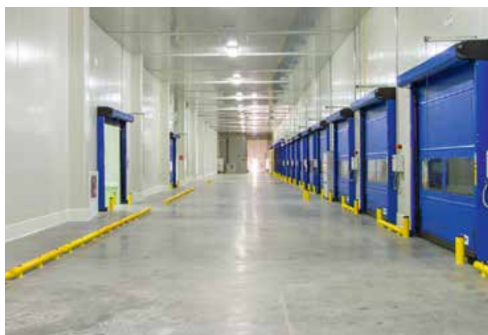
Guardrails for aisle
