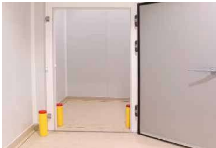
Bollards for protection of shelves and doors
